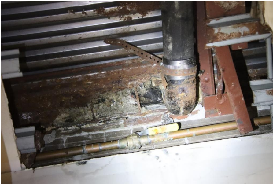
Figure 13. Deteriorated composite deck with section loss around the second floor bathroom drain pipe
