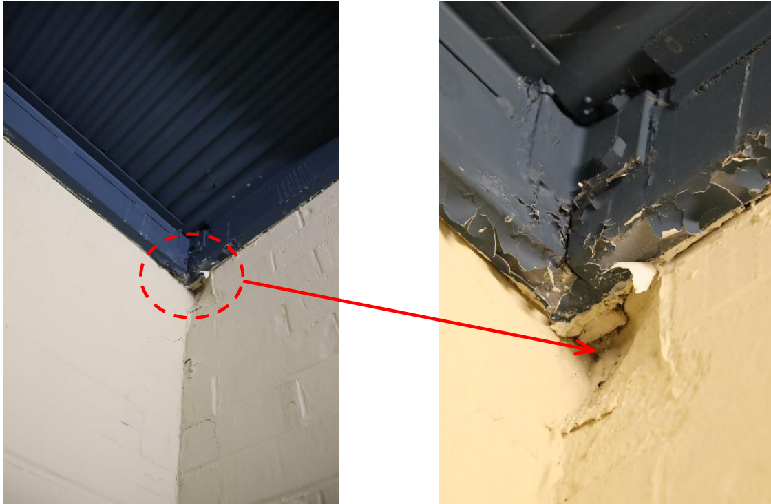
Figure 28. Overall and close-up views of spalled CMU below steel girder bearing in the east stairway, at mid-landing between first and second floor
