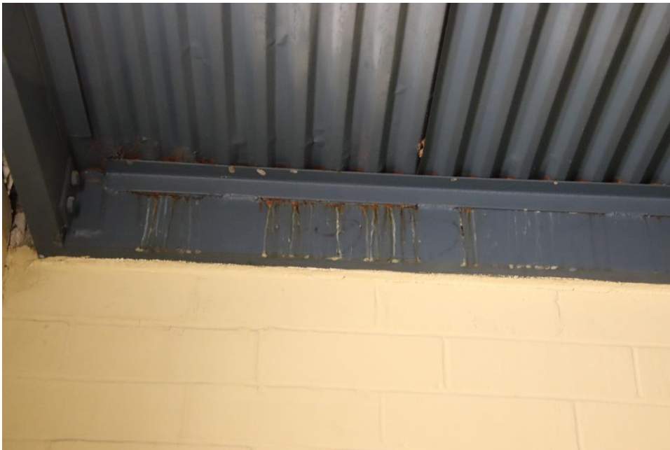
Figure 27. Surface corrosion present on the underside of the sixth floor stairway landing
