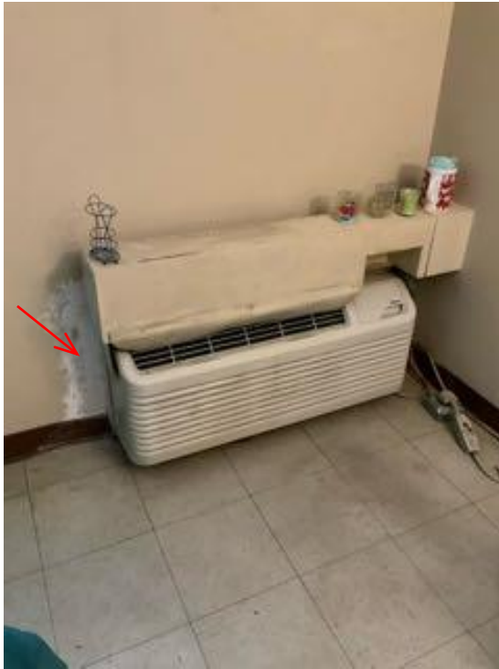
Figure 23. Water damage around A/C unit typ.
