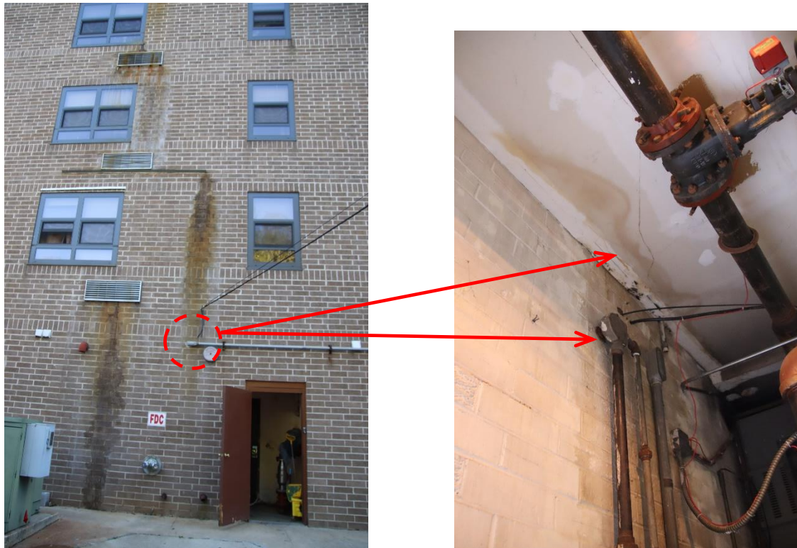
Figure 16. Leaks observed in the mechanical room (exterior and interior side of wall), north elevation
