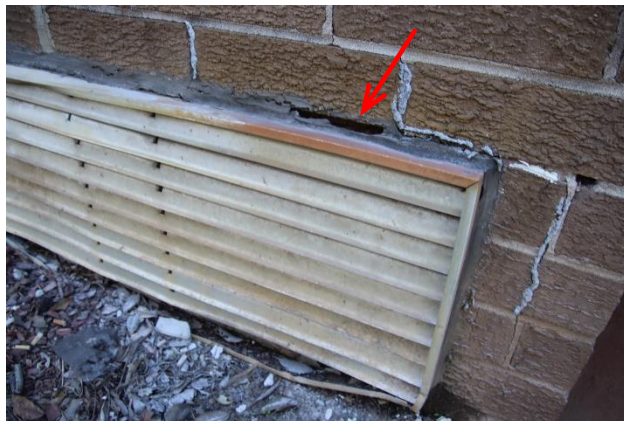
Figure 44. Exploratory opening #4. Sealant and compressible joint filler present over corroded steel lintel above A/C sleeve
