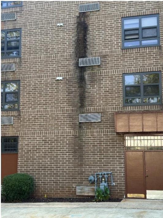
Figure 19. Staining at brick masonry at the east end of the north elevation below A/C
