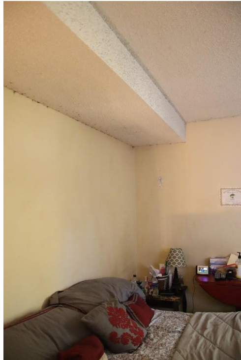
Figure 24. Mold observed on walls in Unit 201
