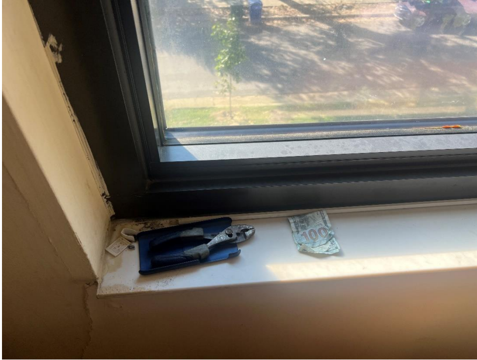
Figure 8. Water damage at the base of the window, Unit 208
