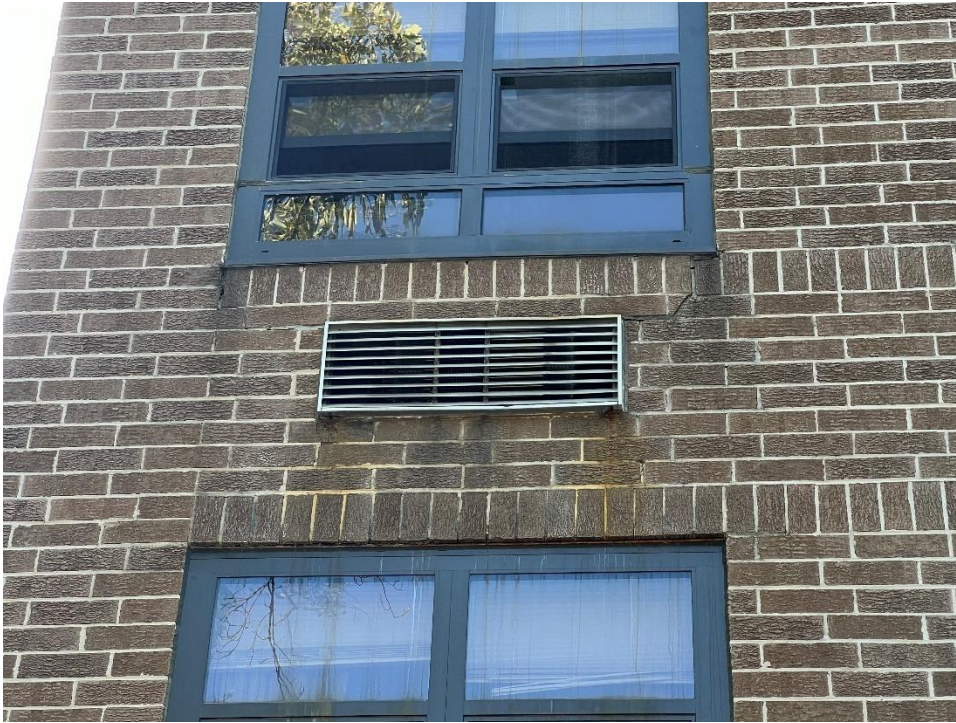
Figure 18. Cracks in brick masonry and corrosion build up at embedded steel lintels above A/C sleeves on the east end of the north elevation
