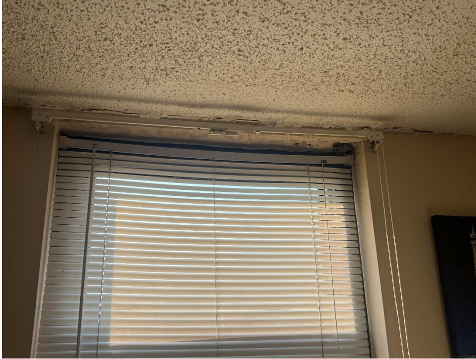
Figure 16. Water damage present above the bedroom window, Unit 502
