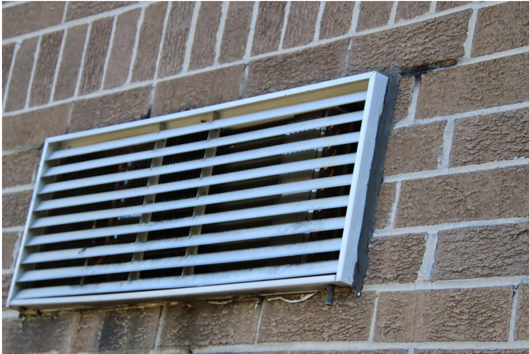
Figure 34. Deteriorated sealant around A/C louvers
