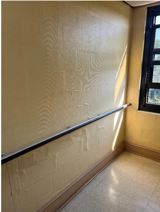
Figure 17. Step crack in the CMU wall at fifth floor hallway
