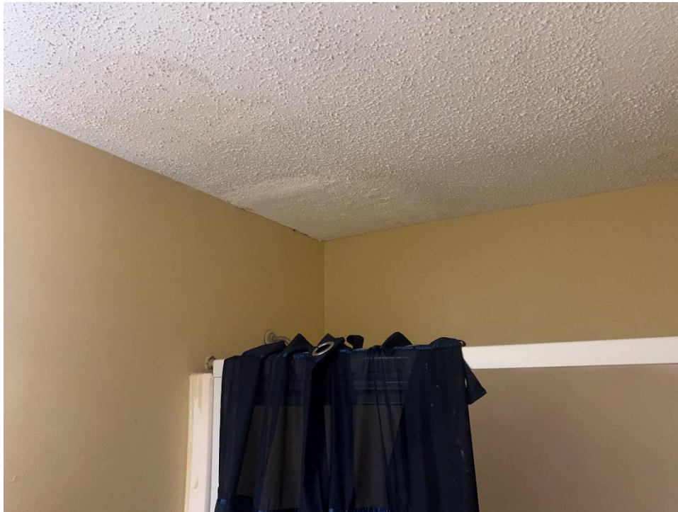
Figure 11. Water staining is present adjacent to repaired area at the bathroom's ceiling, Unit 404
