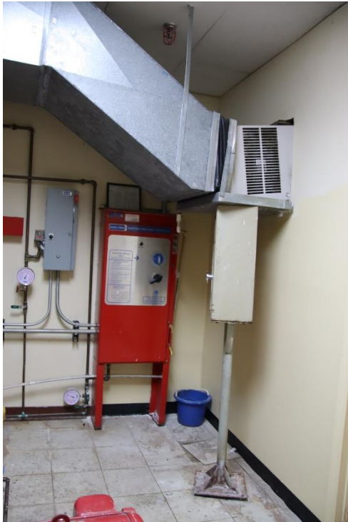
Figure 26. Improvised duct support in the mechanic room adjacent to laundry room
