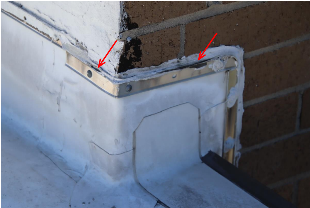
Figure 39. Debonded sealant at termination bar
