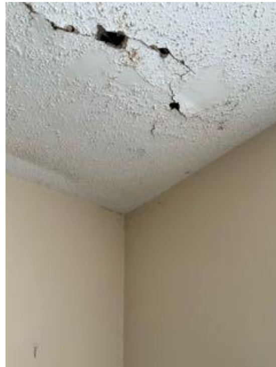
Figure 22. Damaged ceiling due to water infiltration two feet from the exterior wall, Unit 508
