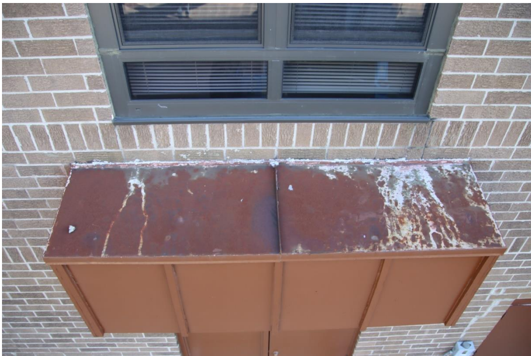
Figure 35. Deteriorated sealant between canopy and exterior wall and worn out paint at the top of the canopy
