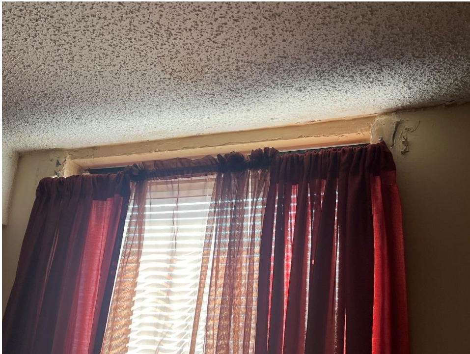
Figure 13. Water damage above the window in Unit 410
