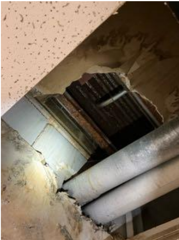
Figure 14. Corroded underside of the second floor composite deck by the exterior wall at the southeast corner of the building
