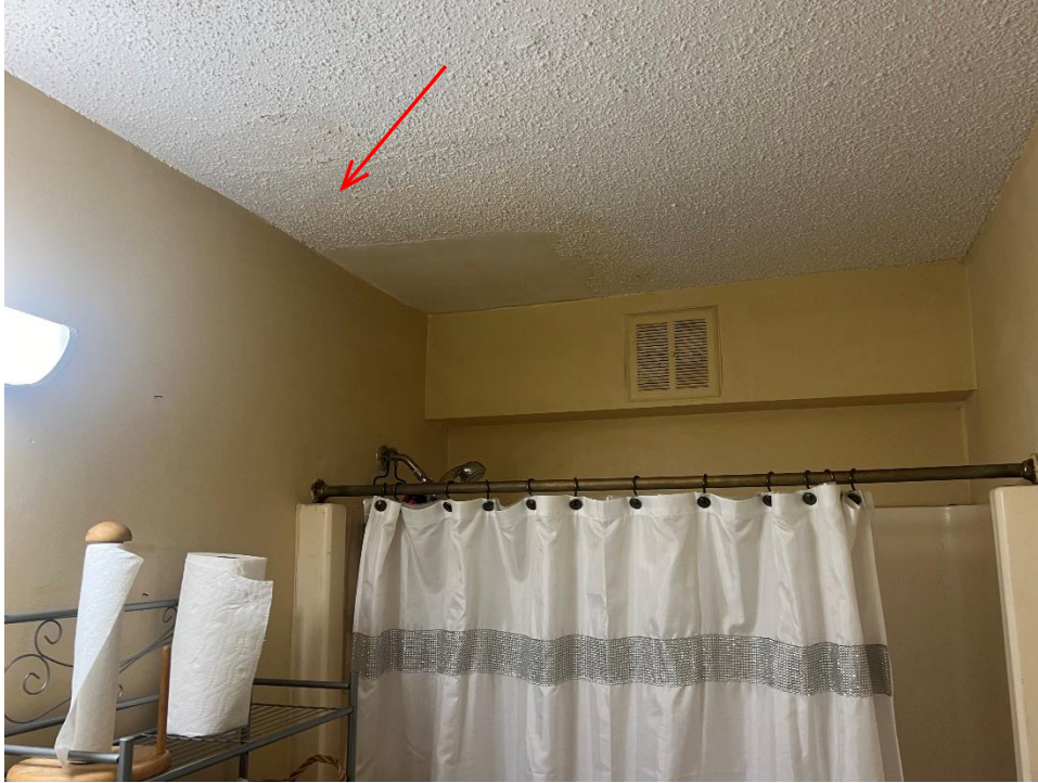
Figure 10. Water staining is present adjacent to repaired area at the bathroom's ceiling, Unit 303
