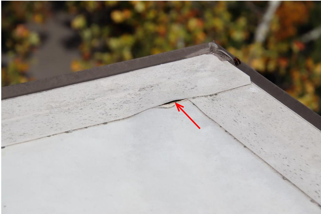
Figure 38. Open seam
