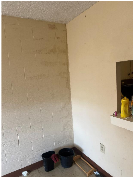
Figure 9. Water damage at the interior corner of the CMU partition wall
