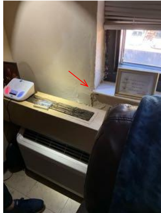
Figure 20. Water damage around window in Unit 303
