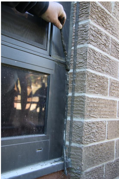
Figure 43. Exploratory opening #3. Removed sealant. No compressible joint filler present between window frame and brick masonry
