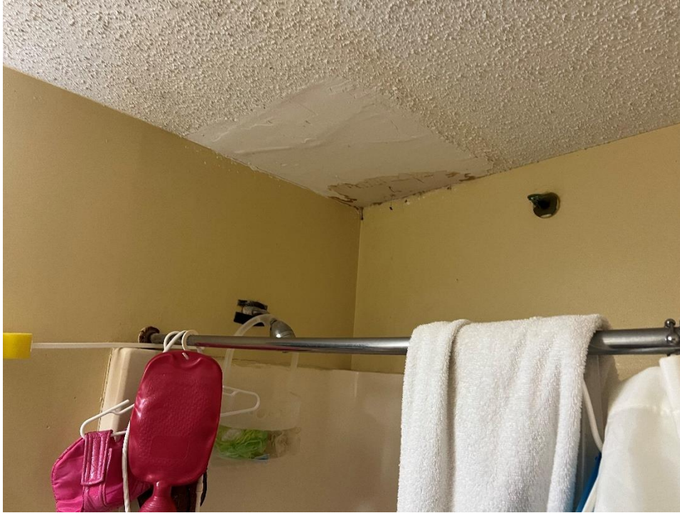
Figure 14. New water leak adjacent to the repaired area of the bathroom ceiling, Unit 501
