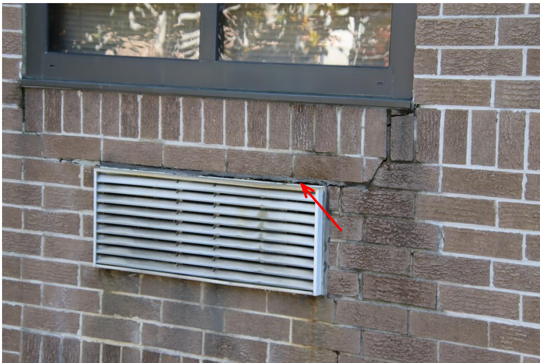
Figure 31. Corroded steel A/C lintel with packed rust
