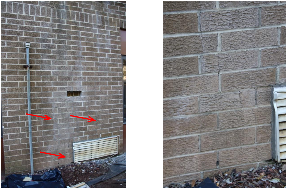
Figure 29. Overall and close-up views of cracks observed in the north exterior wall.
