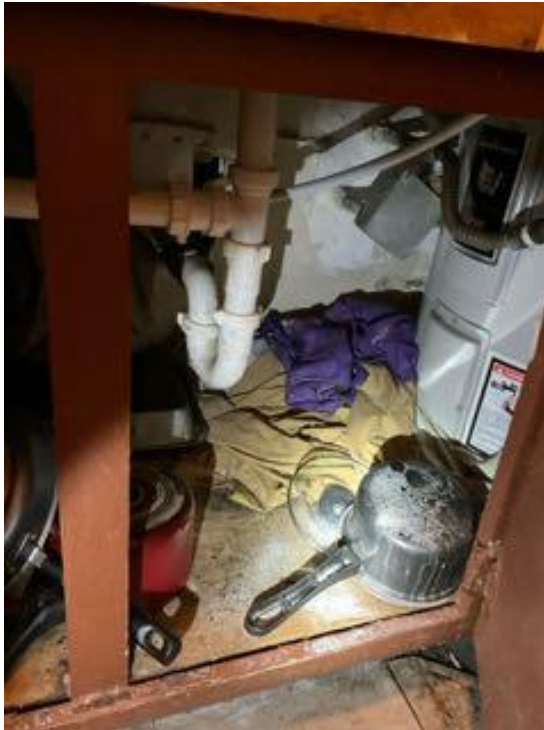
Figure 19. Water damage inside kitchen cabinet from past leaks
