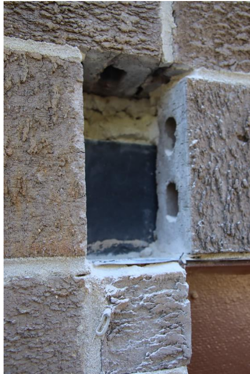
Figure 42. Exploratory opening #2. Overall and close-up views of PVC flashing over steel lintel
