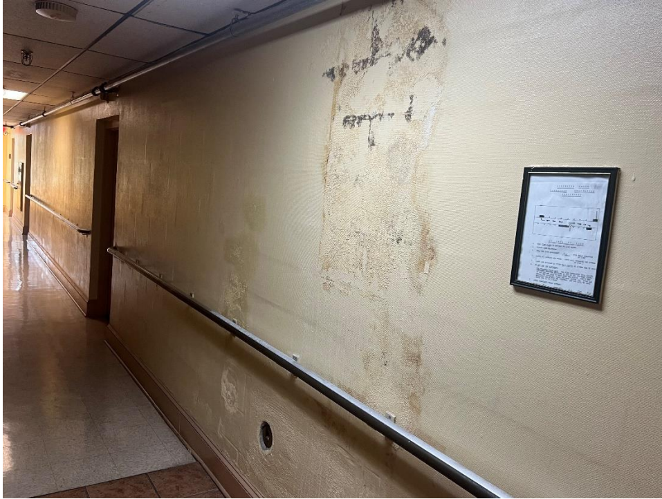
Figure 12. Water damage in the wall at fourth floor hallway
