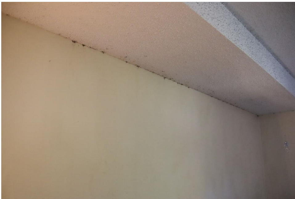
Figure 25. Mold present along the duct and in the wall below it in Unit 201
