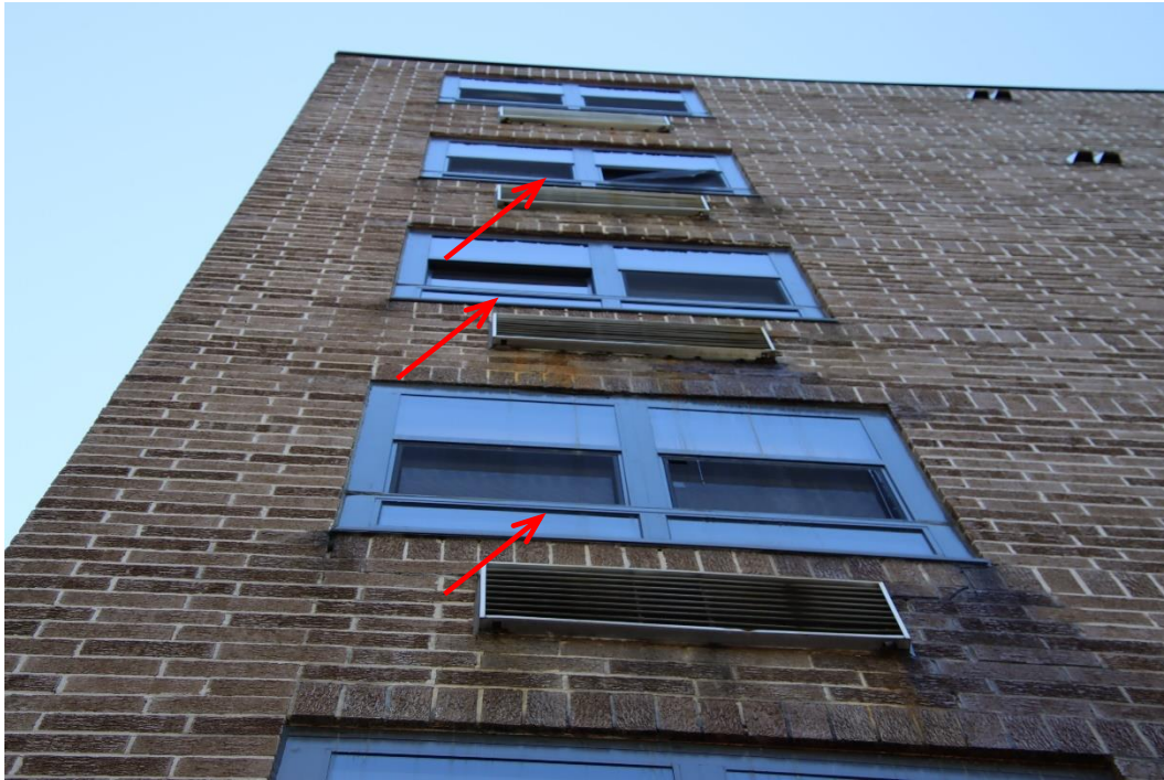
Figure 36. Windows appear distorted out of plane, pushed inward above bottom sash
