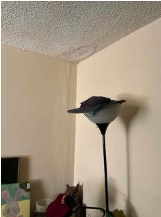
Figure 21. Water damage in drywall at ceiling by the exterior wall, Unit 218
