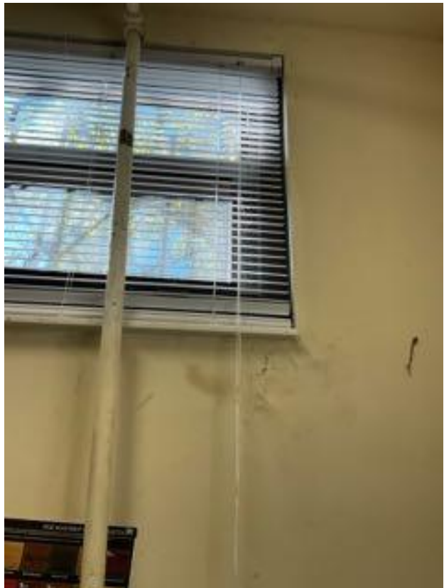
Figure 15. Water damage on the east wall in the office by the south community room, first floor
