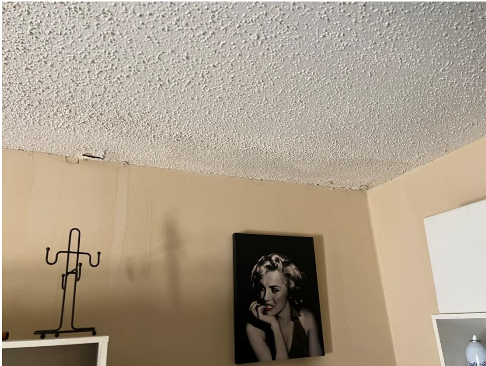
Figure 15. Stains from water leak along the edge of the ceiling against the exterior wall, Unit 502
