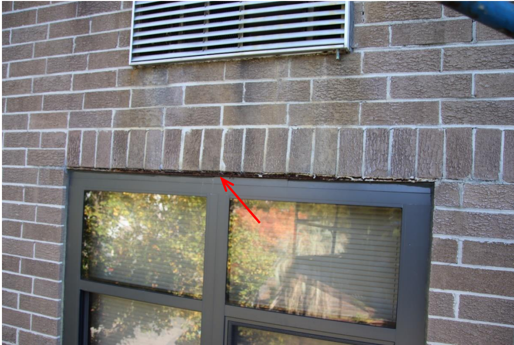
Figure 30. Corroded steel window lintel with packed rust
