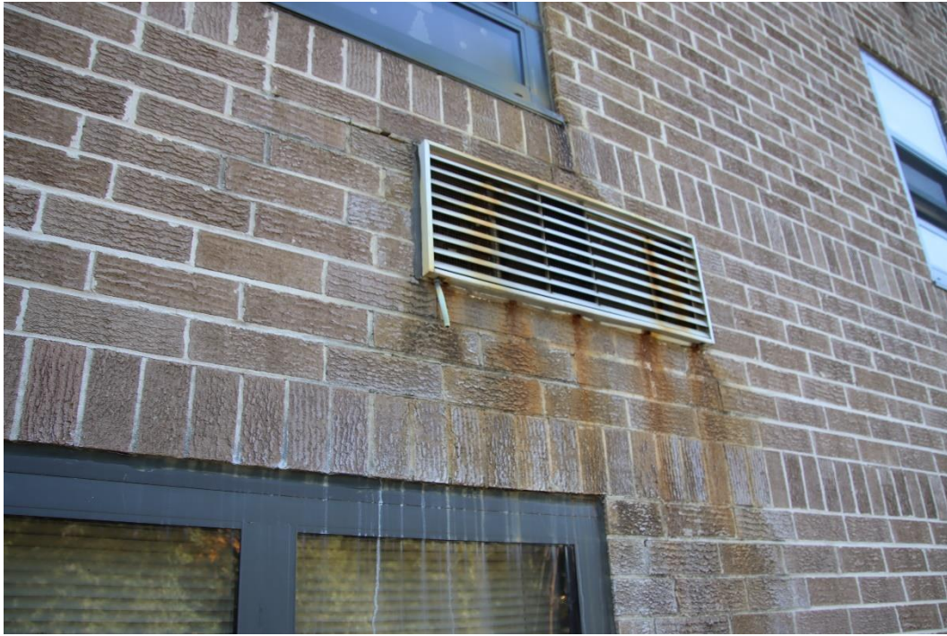
Figure 32. Weeps at A/C sleeves and rust stains below them
